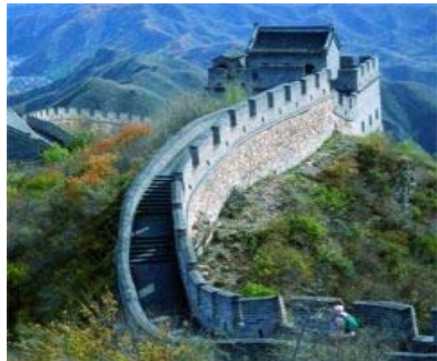
The Construction of the Great Wall.
